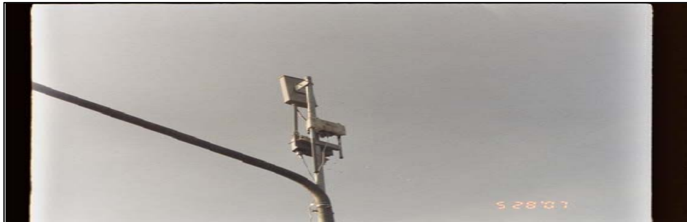
Figure V-11. ES520 and Mesh Dynamics root APs configuration at Mae Ngat Dam, Thailand 2007.
